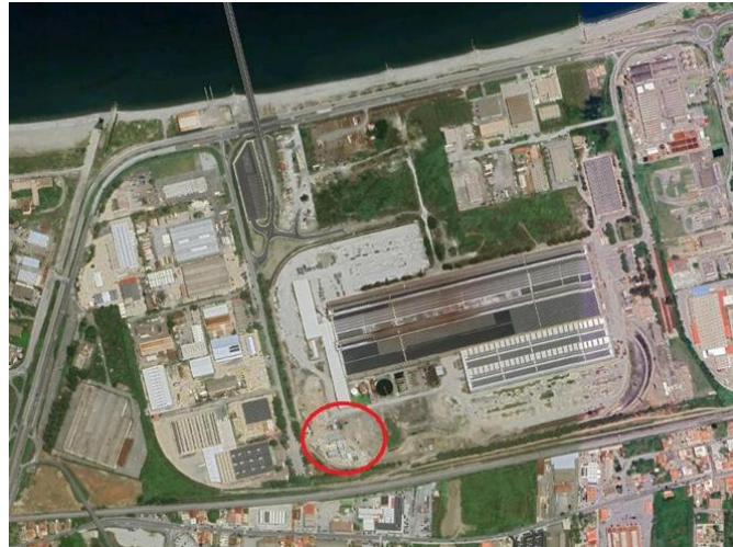
Figure 7 Aerial view of the area involved in the project
