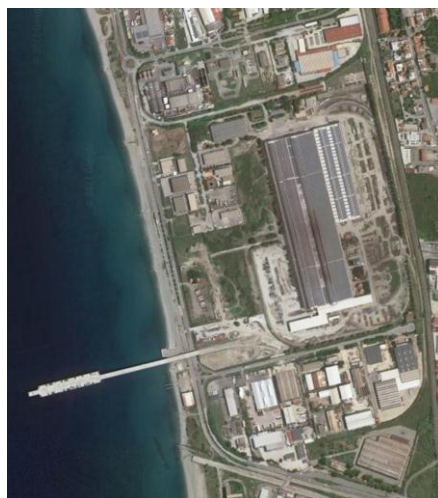
Figure 1 View of the Duferco industrial area
