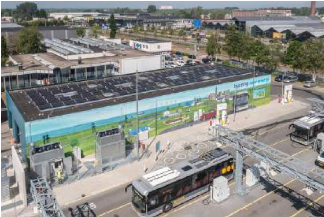
Figure 19. QBuzz filling station (Fuel Cell Electric Buses, 2021)
